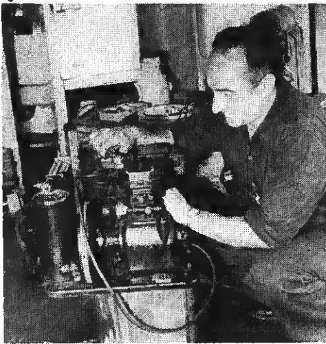
5 Removing head bolts on unit (Kelvinator). Compressor is thoroughly reconditioned.
